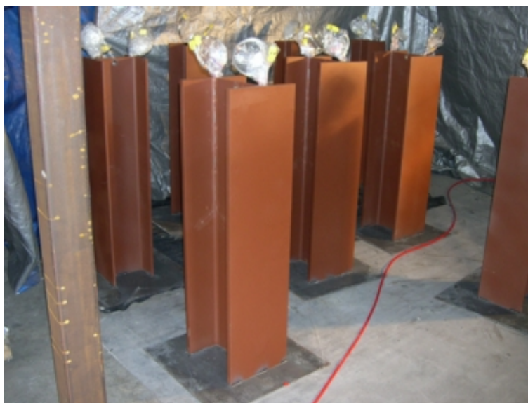
Columns Ready to Spray
