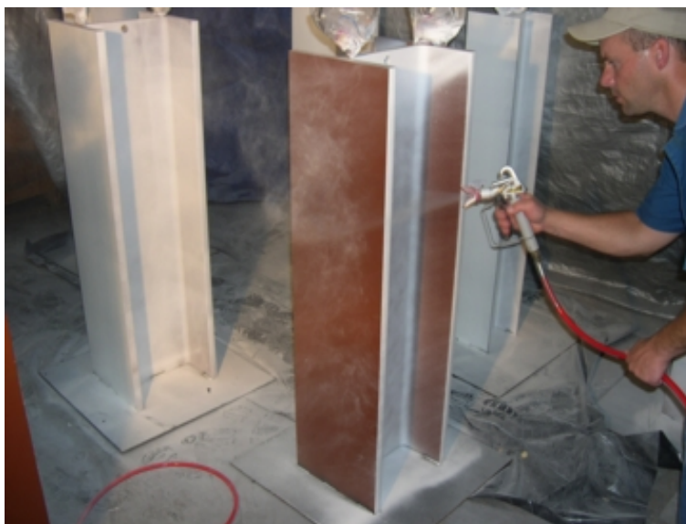
Applying the Coating
