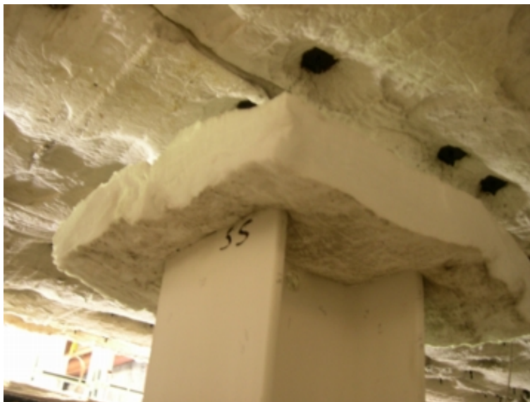
Column Tops Insulated with Ceramic Blanket and Pressed Against Furnace Lid
